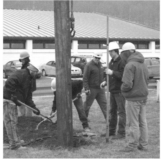
DCEC Linemen donate their time to help SUNY Delhi students in the Electric Utility Operations class set poles on campus that are used as part of the students training.
