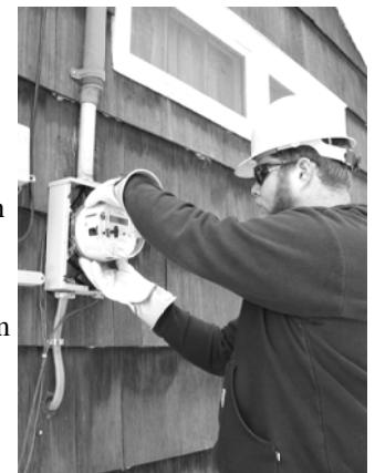
DCEC employee Ryan Sullivan installing a new AMI meter
