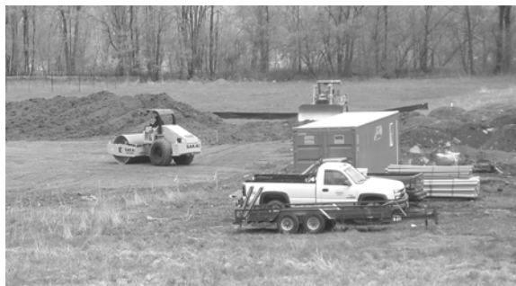
Breaking ground at the Delaware County Solid Waste Management Center
