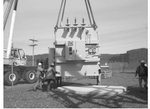
New transformer being placed on concrete pad
