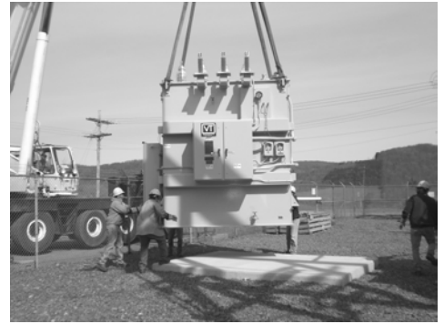
New transformer being placed on concrete pad
