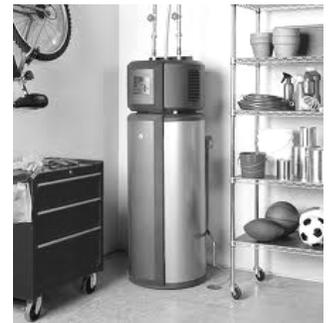
*Example of a heat pump hot water heater*
