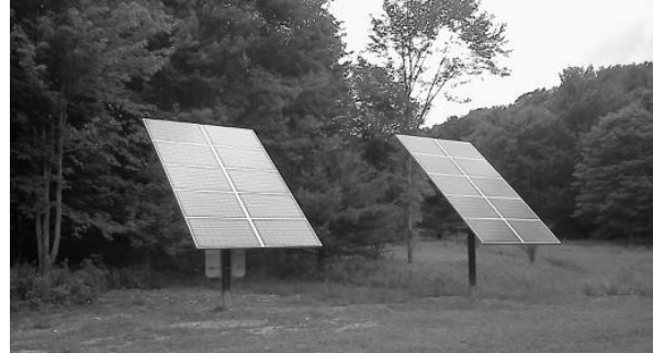
Completed Solar/PV project at member Thomas Daly's home in Harpersfield,
