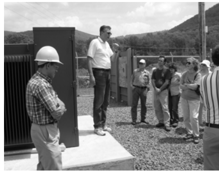
DCEC CEO, Greg Starheim & Engineering Technology Manager, Paul DeAndrea speak to participants of Cornell Cooperative Extension’s 29th Annual Spring Housing Tour at the Delaware County Landfill Waste-to-Energy Project
