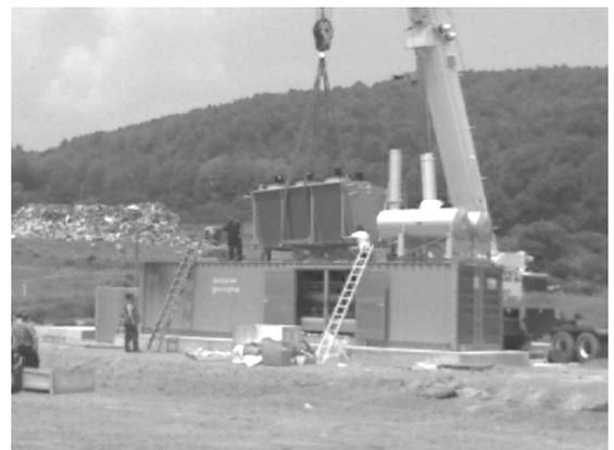
*Installing the radiator on the new engine-generator*
