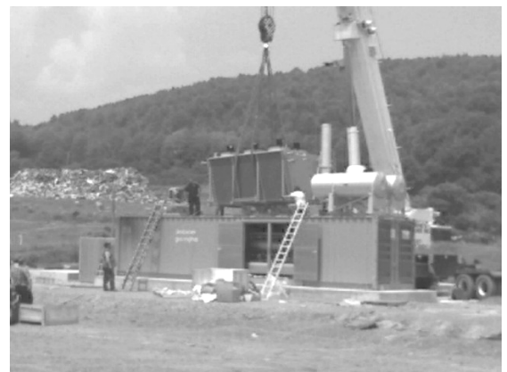
Installing the radiator on the new engine-generator
